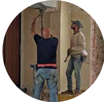
HOUSE RESTORATION - VILLAT
